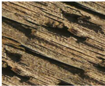
The defects of "The Power of Orient" building roof. Magnified section of the rotten wood under leakages from the roof. Patching and resurfacing of rotten wooden beam by KF-H spray with consequent layer application by trowel.
