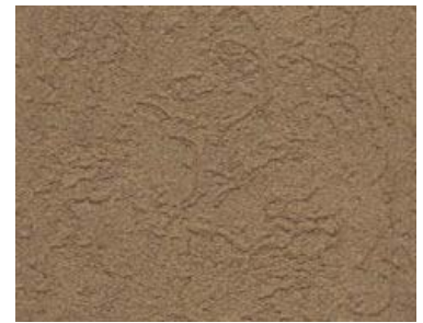
The defects of "The Power of Orient" building roof. Magnified section of the rotten wood under leakages from the roof. Patching and resurfacing of rotten wooden beam by KF-H spray with consequent layer application by trowel.
