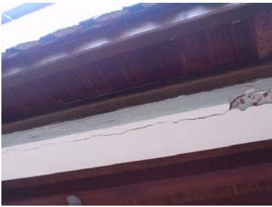
The defects of "The Power of Orient" building roof. Magnified section of the rotten wood under leakages from the roof. Patching and resurfacing of rotten wooden beam by KF-H spray with consequent layer application by trowel.
