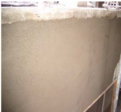
KF-F applied on a kiln foundation under temperature 185°F or 85°C (Poland).
