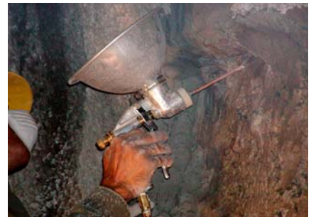
"Welding of Concrete" with KF-C stops any leaks and resurfaces concrete defects.
