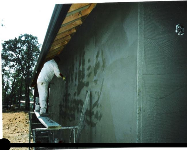
Mix design is simple, as shown below. Batch was prepared by pale-shovel measurements, where a Coca-Cola can represented 1 pound of KF-A.
