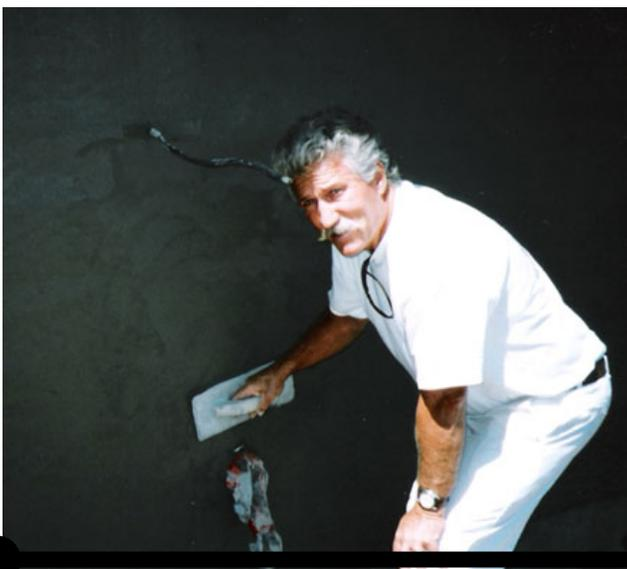
Mortar mix with added KF-A has self-reviving workability – keep mixer rotating and your mix will be workable and finishable as long as application goes.
